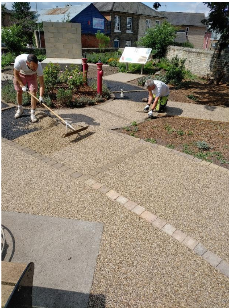
2 August 2019 – Final coat of resin bound aggregate applied over the top of asphalt.
