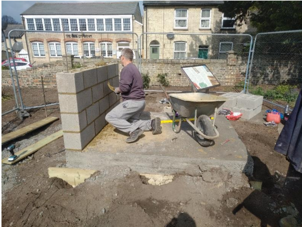
12 April 2019 - Blockwork being laid on top of concrete base to form the back of the structure
