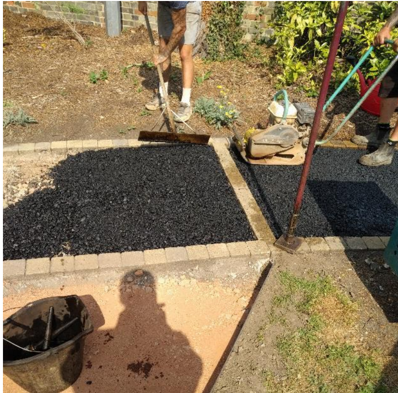
25 July 2019 – asphalt applied over hardcore ready to take final surface
